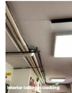
Interior ceiling cracking
